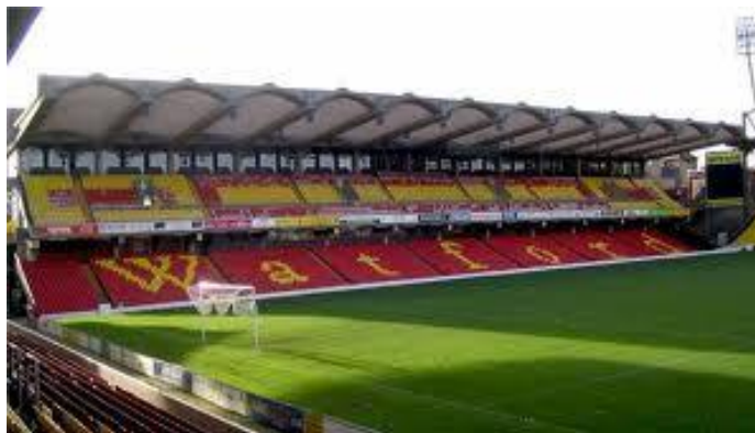
Fig 27: Watford Football Club Stadium
